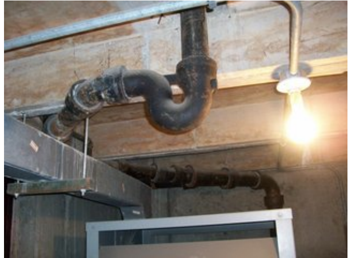
Sanitary drainage Piping
