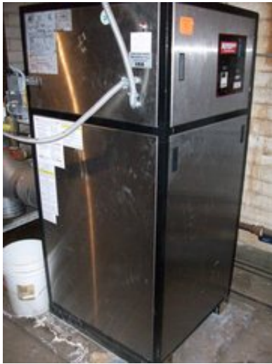
Gas Fired Hot Water Boiler
