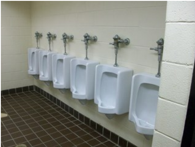
Toilet room fixtures
