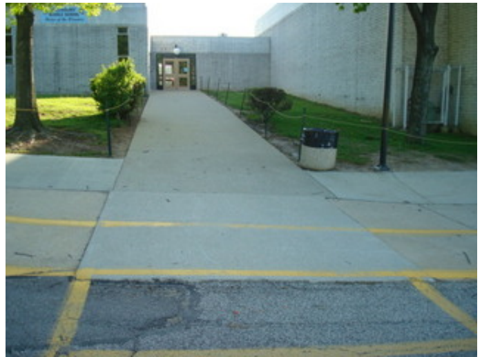
Curb ramp at parking lot
