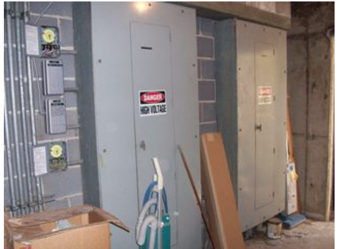
Main Lighting & Heating Panels
