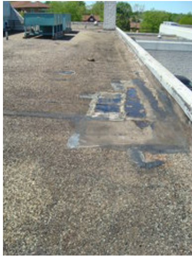
Ponding and patches on built-up roofing
