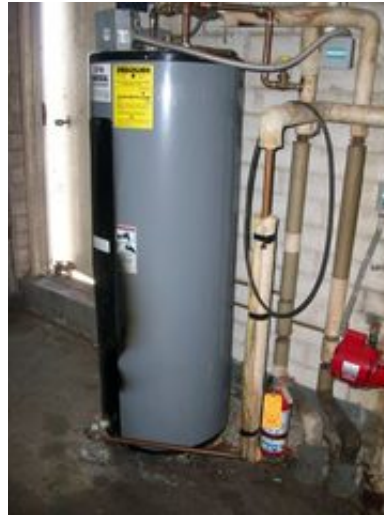
Domestic water piping at water heater
