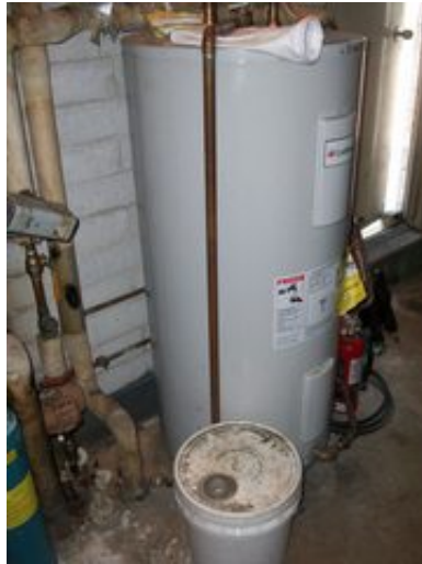
Domestic Water Piping at water heater
