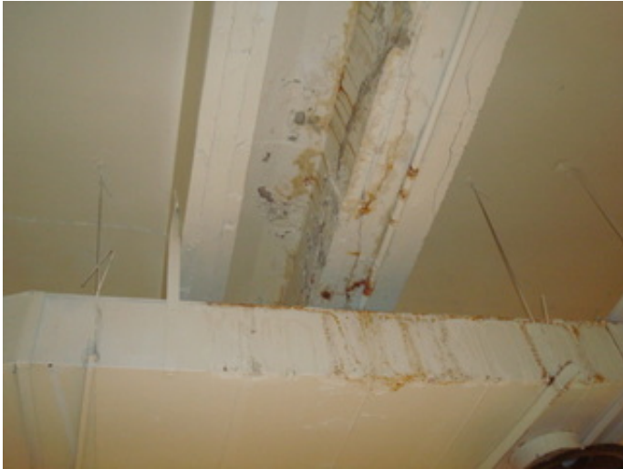
Previous roof leak
