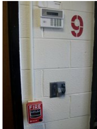
Wall Mounted Security Panel
