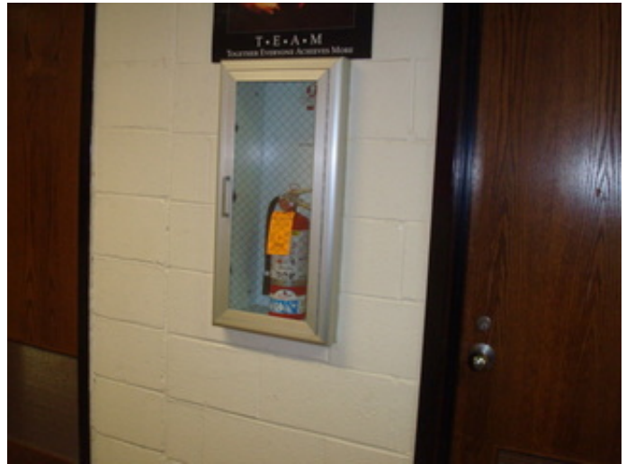
Fire extinguisher cabinet
