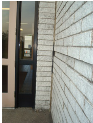
Damaged expansion joint caulk
