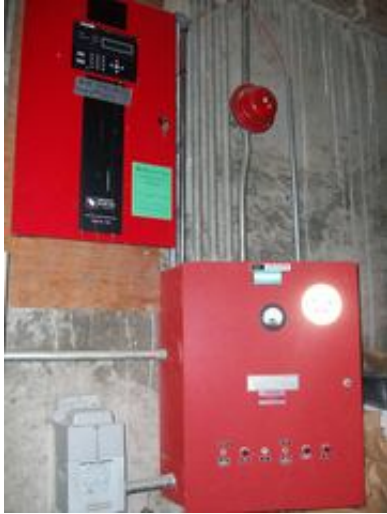
Fire Alarm Panel
