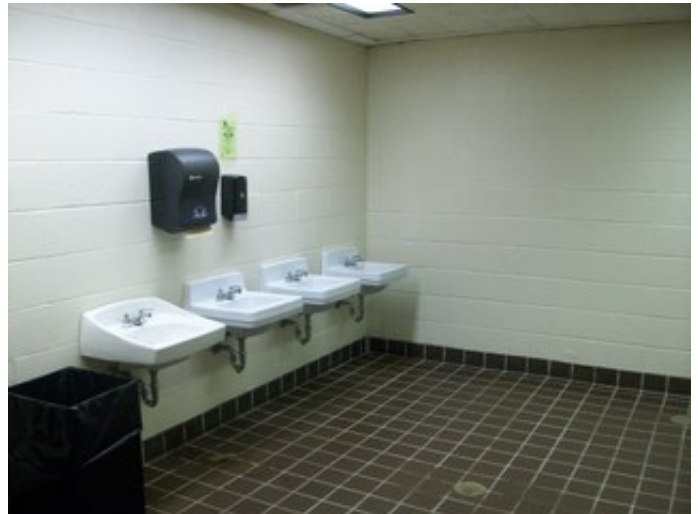
Toilet room fixtures
