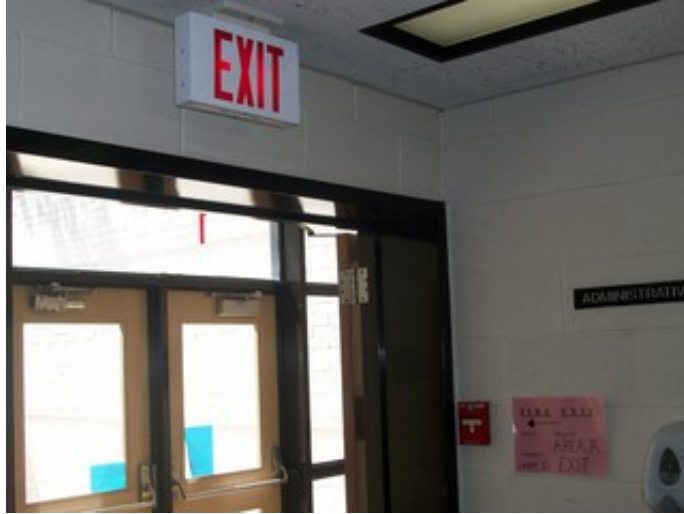
Wall Mounted Fire Alarm Device
