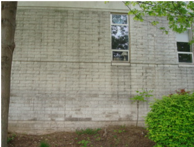
Expansion joint and vertical crack
