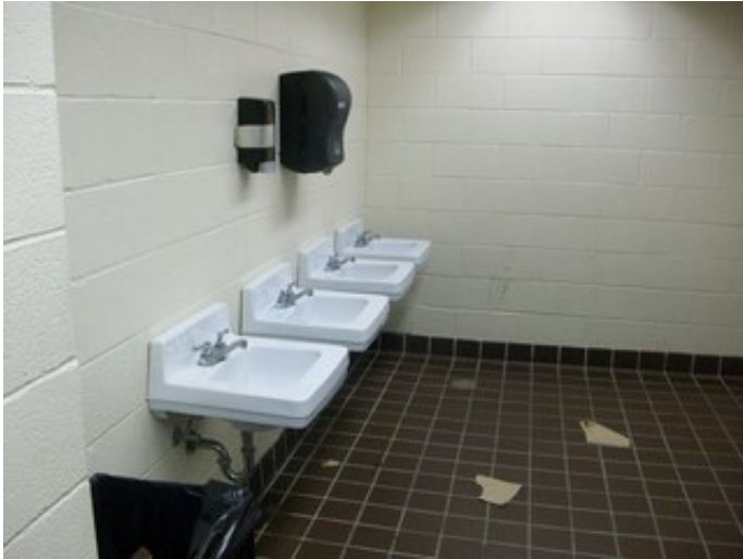
Sanitary piping below sink
