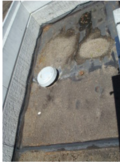
Built-up roofing in poor condition
