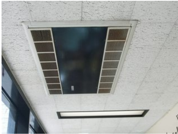
Electric Unit Heater
