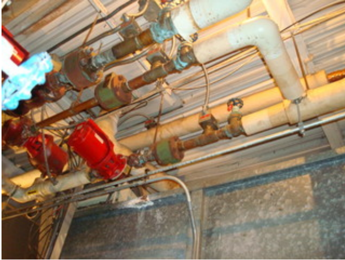
Non ACM pipe insulation
