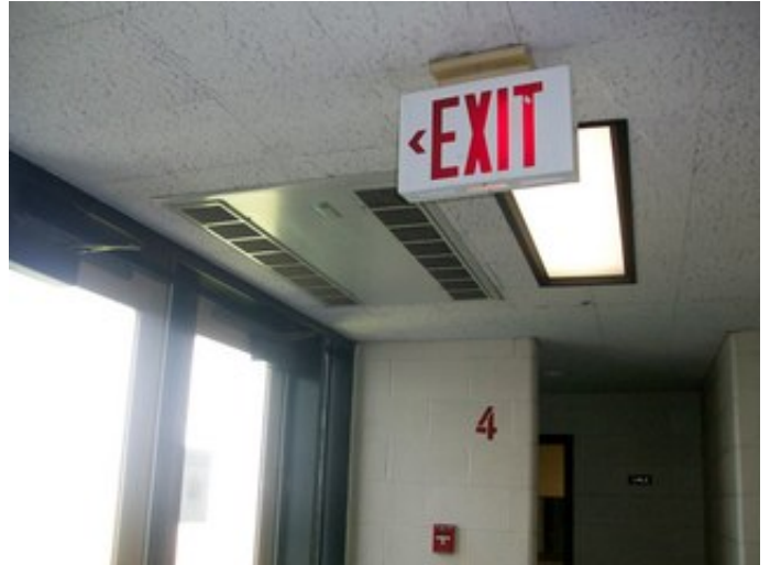
Ceiling Mounted Exit Sign
