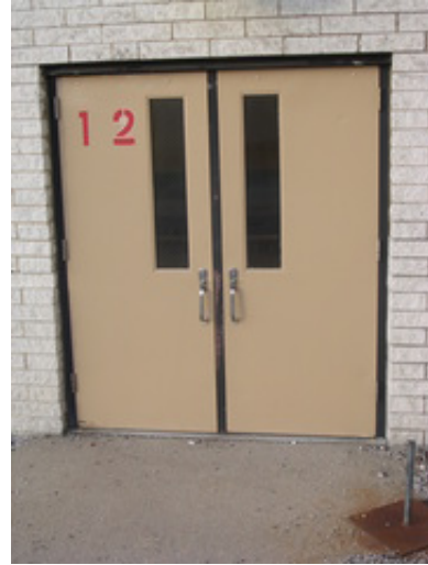
Typical hollow metal door.
