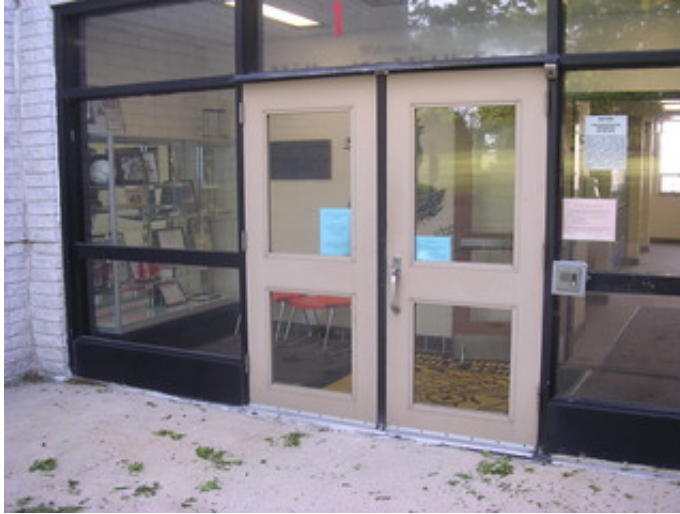
Typical hollow metal entry door.
