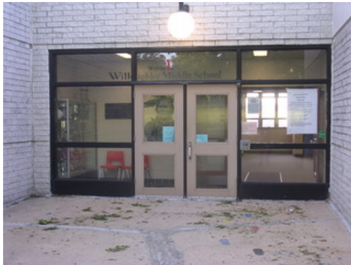
Typical hollow metal storefront system.
