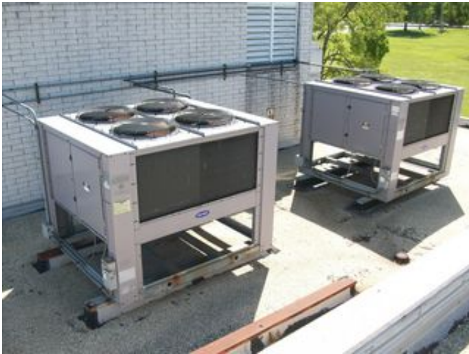
Roof Top A/C And Exhaust Fans
